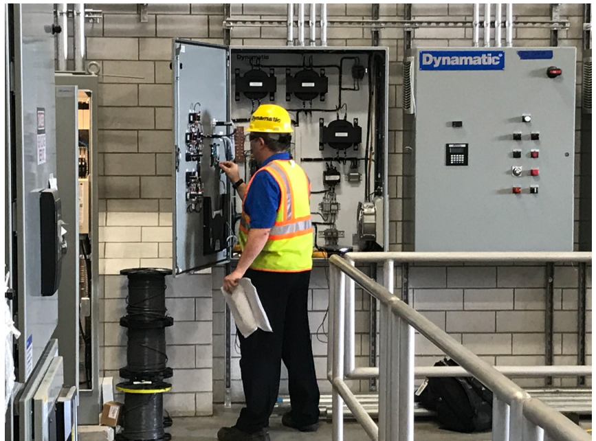
Figure 4 : Completed modified enclosure with customized EC-2000HP Controller
